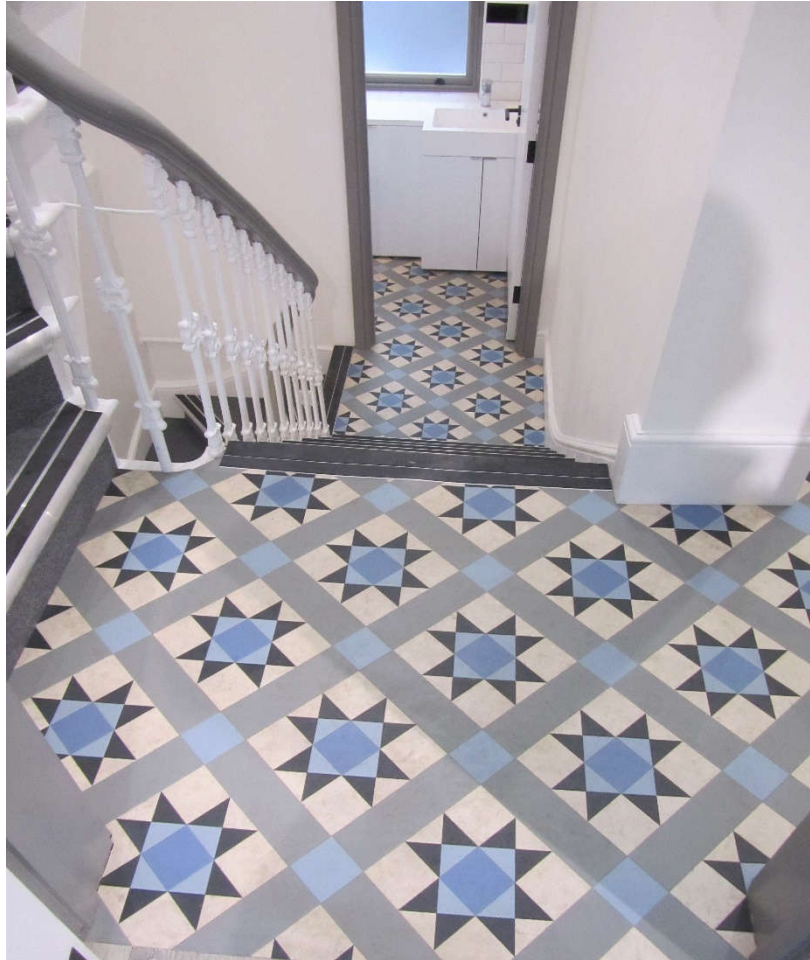
Image above shows Antico flooring to WC, staircase and landings.
