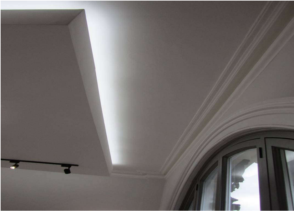
Image on left shows floating ceiling with LED lighting detail
