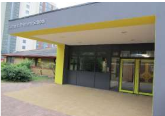
Steel and timber construction to cantilevered canopy
