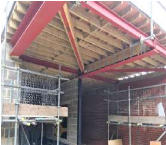
Steel and timber construction to cantilevered canopy
