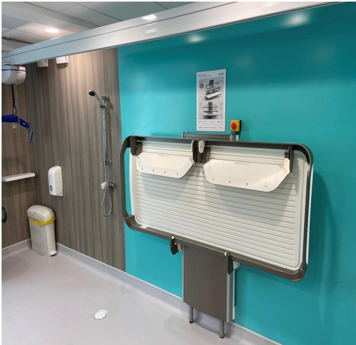
Images show, Astor Bannerman height adjustable changing bench, level access shower area with mixer shower, Arjo Maxi Sky ECS hoist, raised height WC suite with Hewi grab rails and drop down rails supplied by Neville Lumb.
