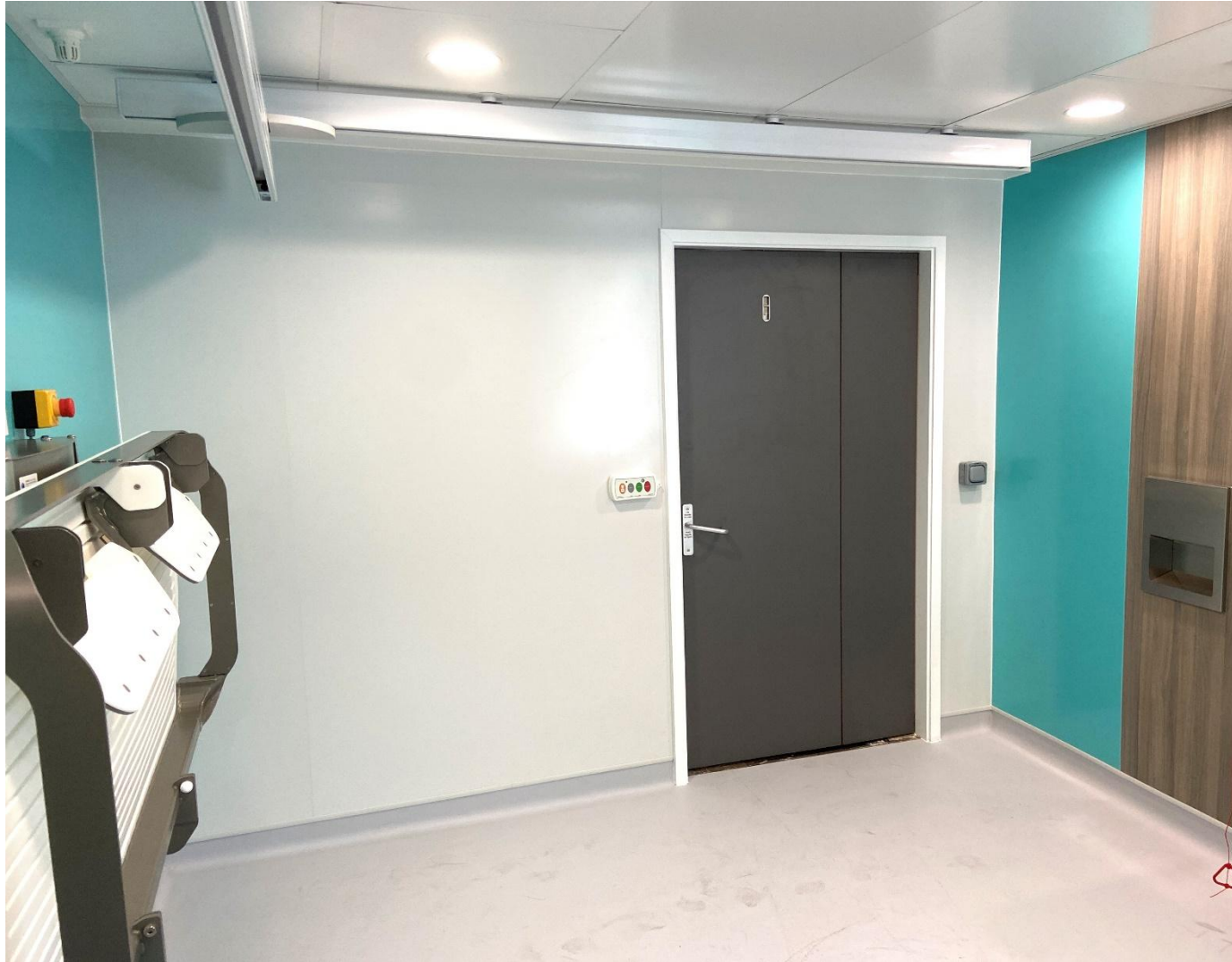
Image above show, Hygienic wheel chair access bi-fold door set with Rada lock by Principle doors, radiant ceiling panels and Ecophon suspended ceiling and nurses call point on right is the ambulant user WC.
