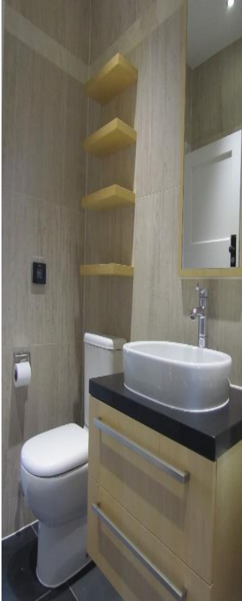
Left/right: images showing completed bathroom and ensuite with fitted bespoke furniture, natural stone surface's, new sanitary ware and lime stone wall tiles.
