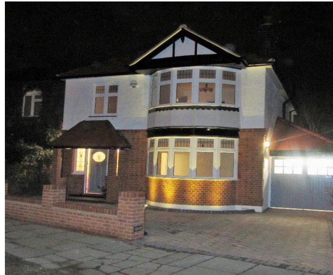
Above: images showing front Elevation during and after construction.
