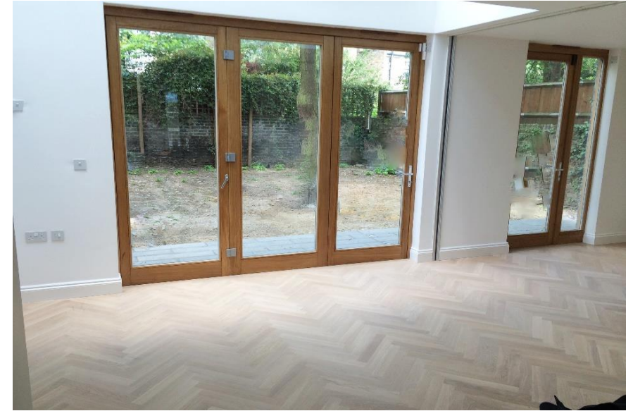
Parquet flooring with under-floor heating was fitted throughout the lower ground floor. Solid Oak folding/sliding doors open up to allow the outside in.
