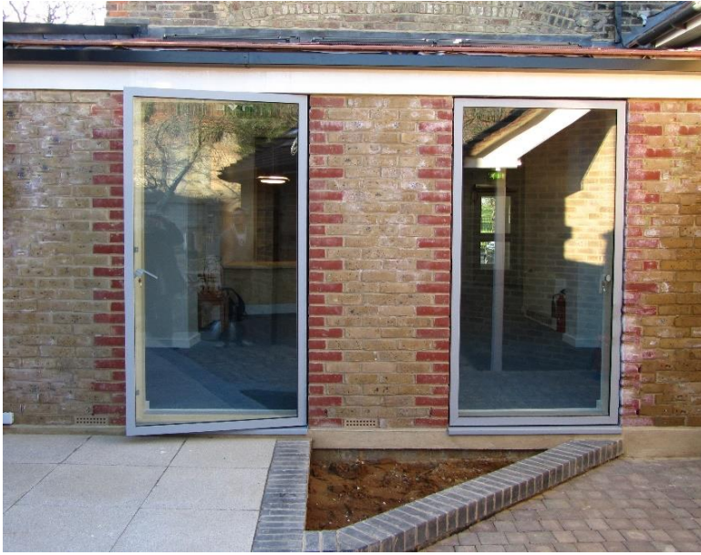
Rear extension with large roof windows to provide Natural light are large high spec doors
